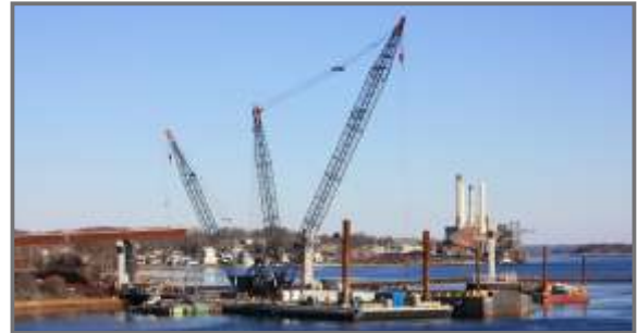
Bridge construction de-watering
