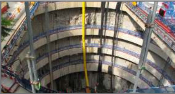
Underground construction de-watering
